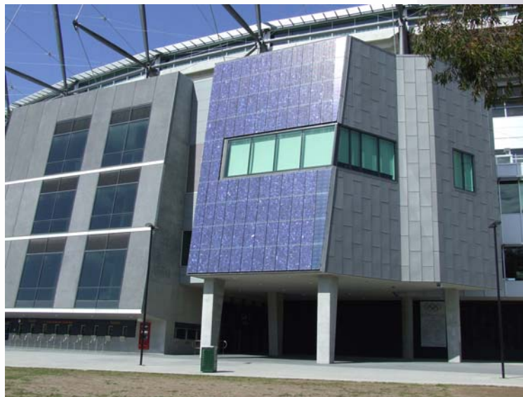
Photo of MCG photovoltaics
