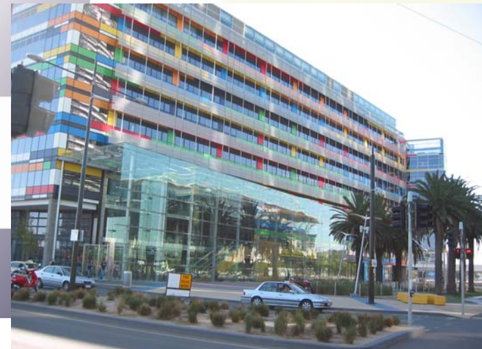
NAB Building Docklands
